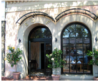
Solé in New Cannan, CT equipped with the innovative hybrid water heating system.
