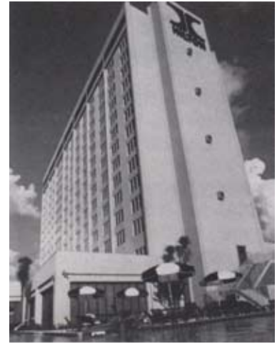
St. Petersburg Hilton and Towers, St. Petersburg, FL
