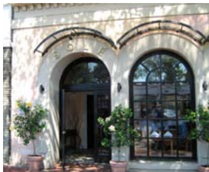
Solé in New Cannon, CT equipped with the innovative hybrid water heating system.
