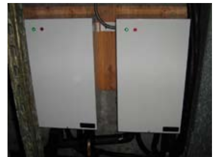
Two Enviro-Pak's generating hot water by recycling wasted heat from the refrigeration system.
